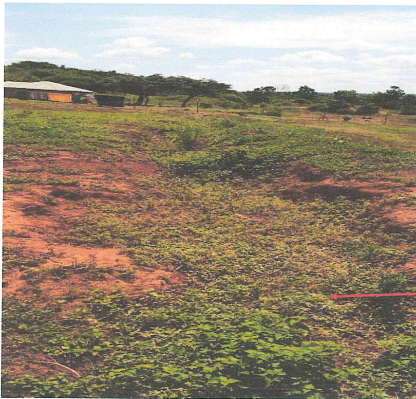
Fig. 2 Drainage for clearing flooding water from the hills behind the college
